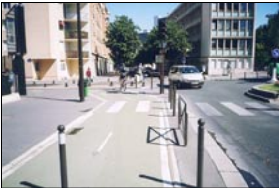
Fencing and bollards for protection
