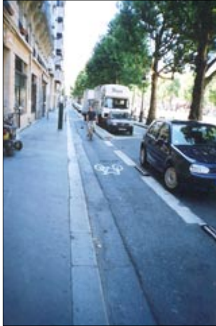
Transition from island separated path to rumble strips
