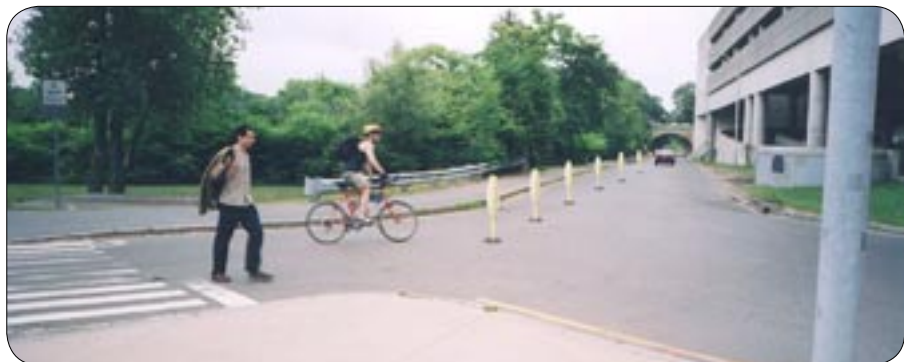
Installation of bollards could better define a pathway within the road right-of-way and separate cars from bicyclists.
