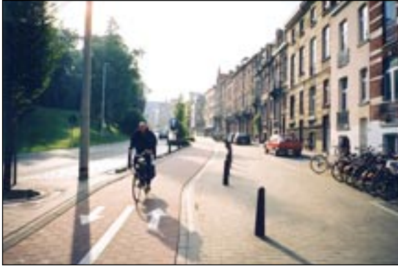
Angled curbs with protective bollards
