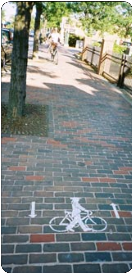
Minuteman bike path stencil used when the path joins city sidewalks. Though not all bicyclists will dismount, the intention is to keep bicyclists on the street side of the sidewalk.
