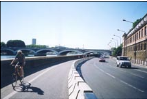
Moveable barrier to accomodate high weekend bicycle use
