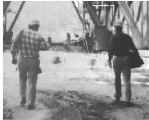
SECURING THE JOB AND CHECKING THE WORK SPACE
